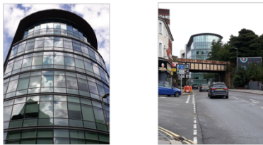
11. Kingsgate at the southern entrance to Redhill
