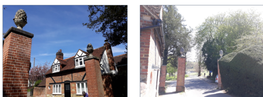
15. Western (Park Lane) entrance to Priory Park
